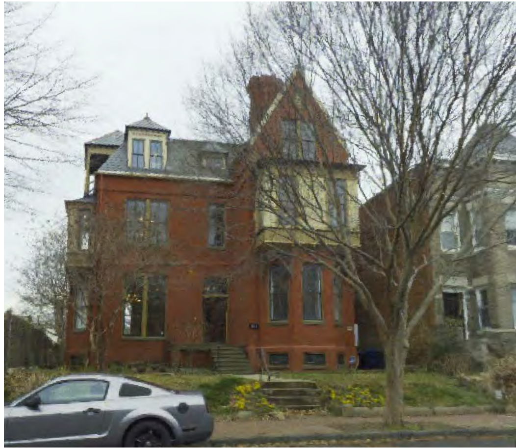
T STREET LOOKING NORTHEAST
