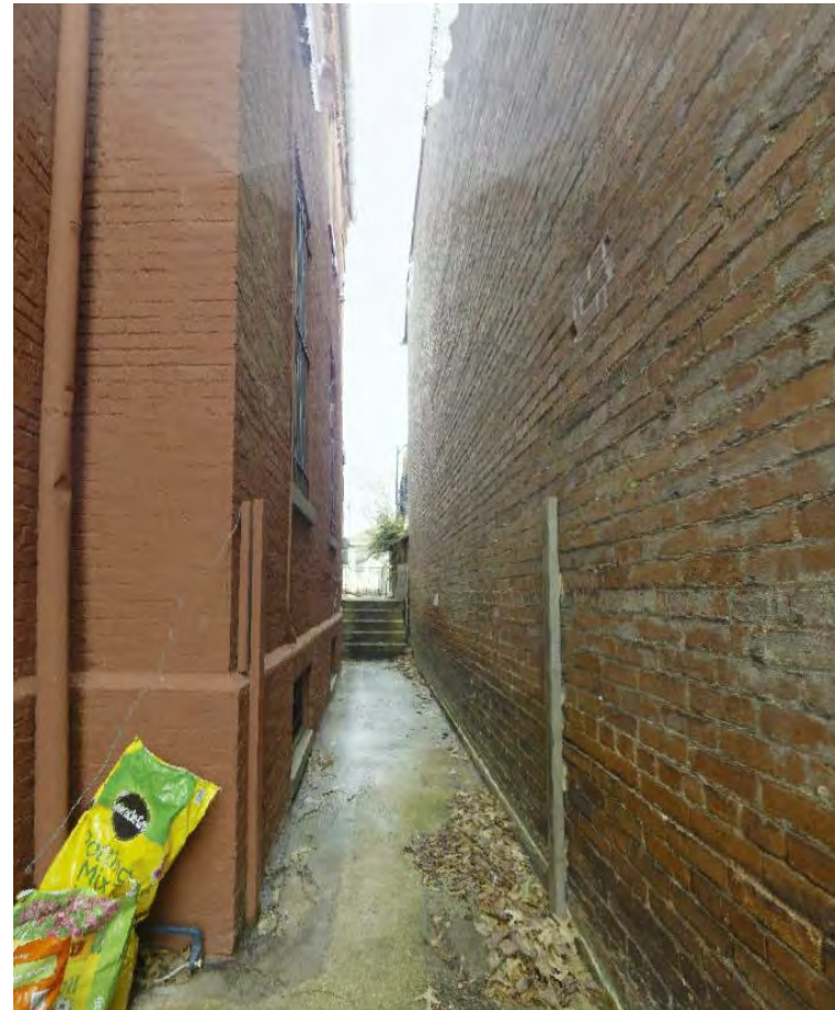
EAST SIDE YARD
