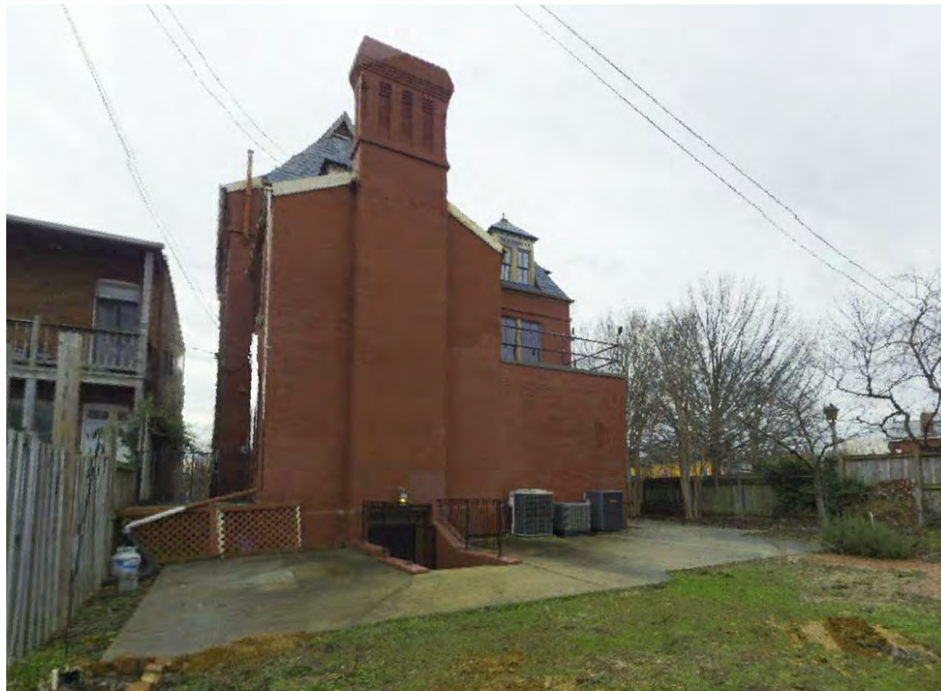
REAR YARD LOOKING SOUTHWEST
